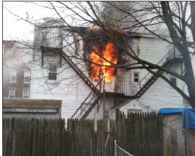
View of the fire building from Side "C" during the initial stages of the fire as Engine 5 was entering from Side "A".
